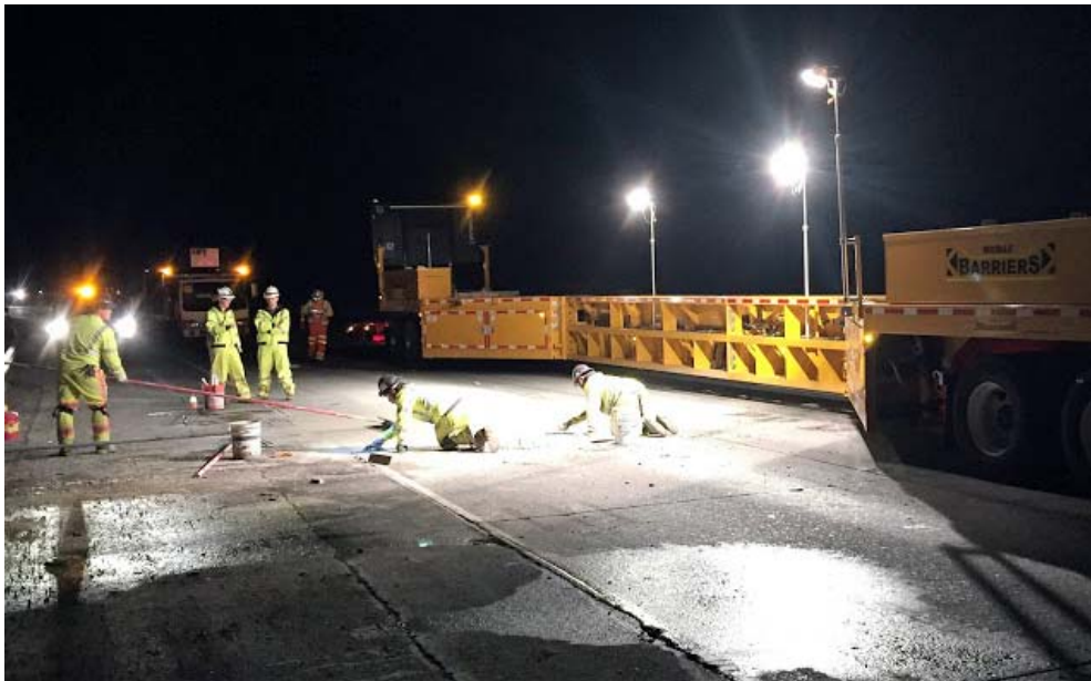
A mobile barrier helps keep our workers safely separated from traffic.
