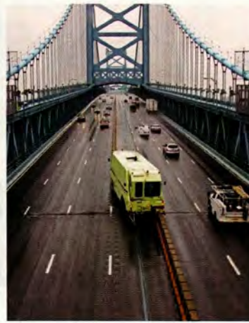
BRIDGING GAPS Movable barriers like the Road Zipper System can quickly add a temporary buffer lane, as on Philadelphia's Ben Franklin Bridge, during construction.
