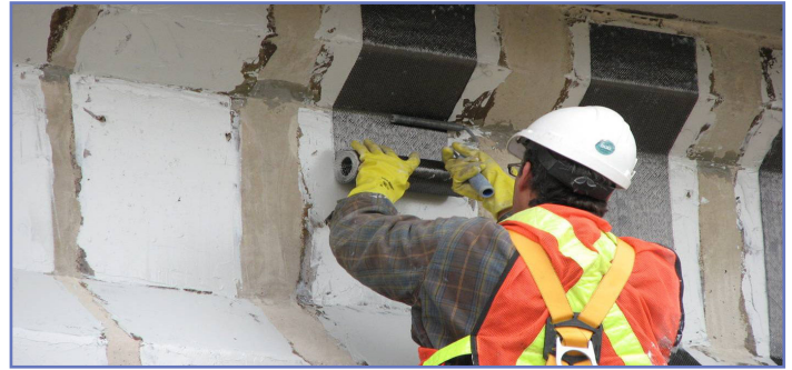
Application of CFRP strips with a roller.
