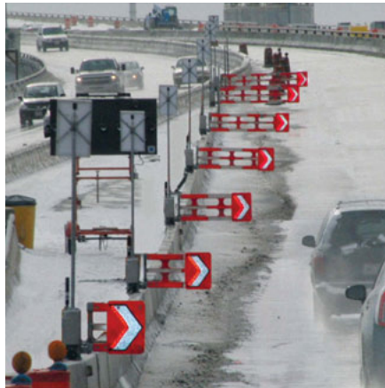
Versilis' SwiftSign automated warning signs and SwiftGate automated gates are being used to increase traffic safety during daily lane closures as work continues on the US$278 million project to replace the entire bridge deck on Hoan Bridge in Milwaukee
