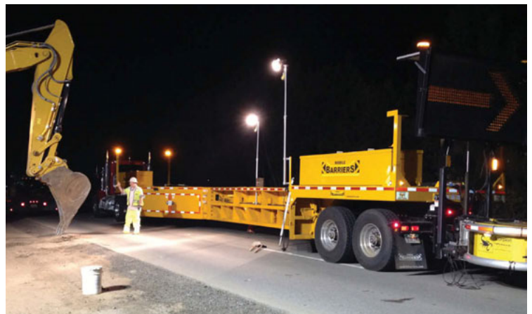
LEFT: The MBT-1 mobile barrier from Mobile Barriers was used by Granite Construction to help complete a full road cut and culvert replacement on the 101 Interstate between San Francisco and Los Angeles ABOVE: The MBT-1 mobile barrier is ready to be deployed by Granite Construction on the Interstate 101 San Francisco-Los Angeles works
