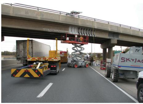
Mobile Barriers 1: The MBT-1 mobile barrier with scissor lift being used near London in Ontario, Canada
